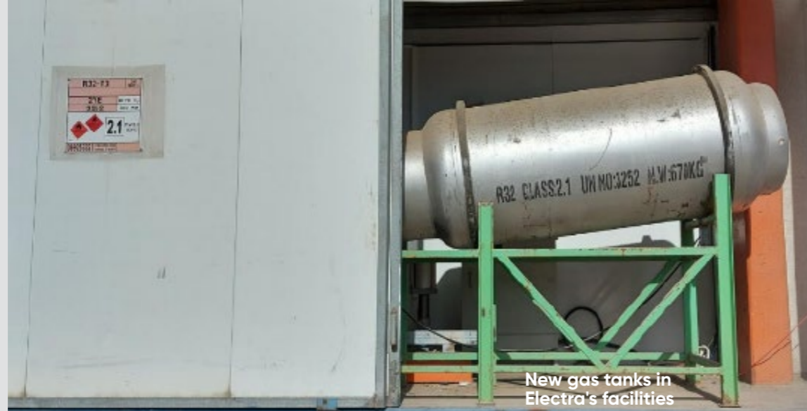
Gas pump system on our production floor
